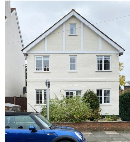
25CR - EXISTING PROPERTY
